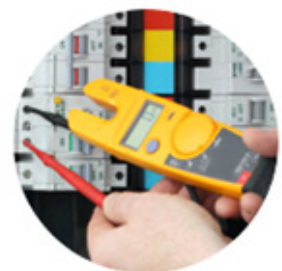
Electrical System Testing and Maintenance
