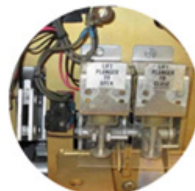
Arc Flash & Low Voltage Safety
