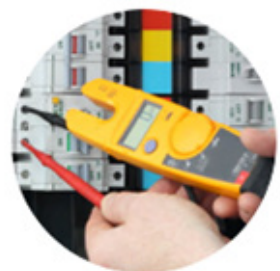
Electrical System Testing and Maintenance
