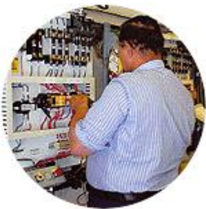
Understanding Low Voltage Electrical Systems
