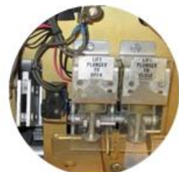
Arc Flash & Low Voltage Safety
